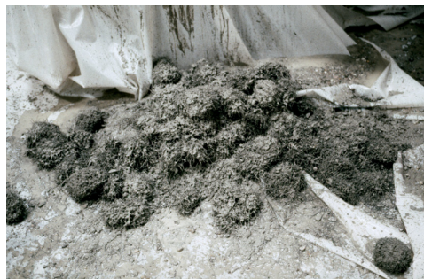
Figure 3: example of typical fibre-balling on site
