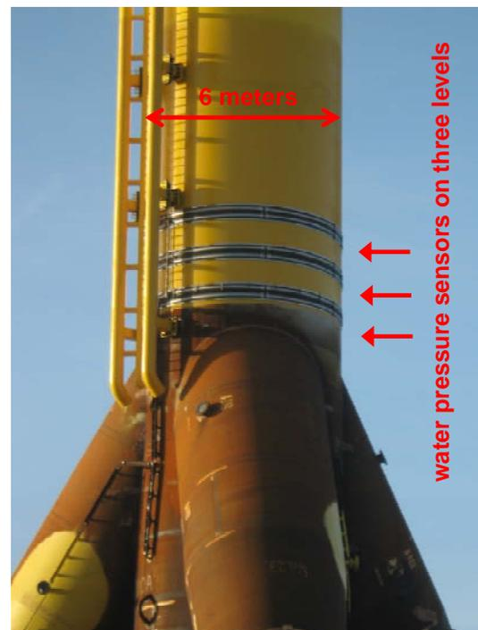
Fig. 1 Multibrud Tripod with measurement system (source: DEWI)
